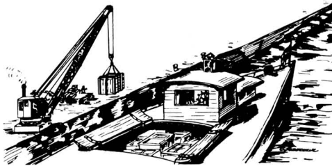
Operating a traveling crane on the river Oder. Eisler was responsible for firing his own boiler.
